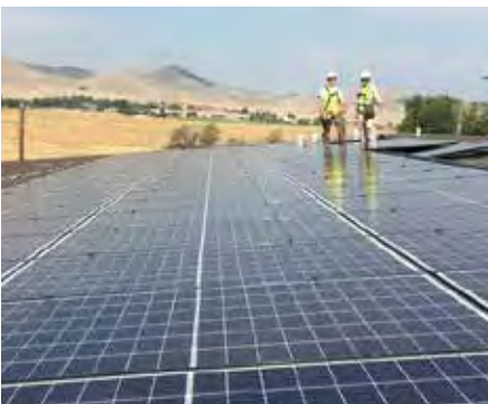
Solar panel installation
